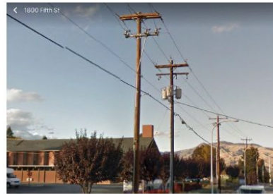
Upgrading existing neighborhood Distribution lines
