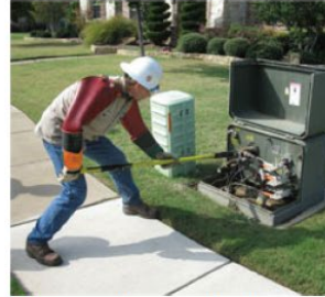
Upgrading existing transformers
