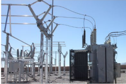
Adding neighborhood Substations
