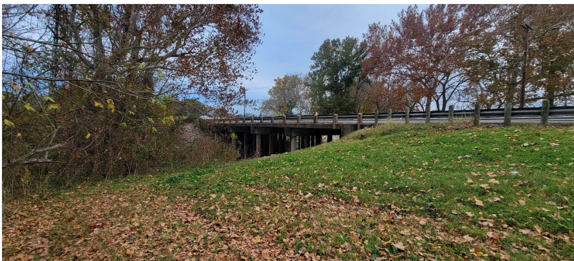
Potential pedestrian passage to Hohlt Park
