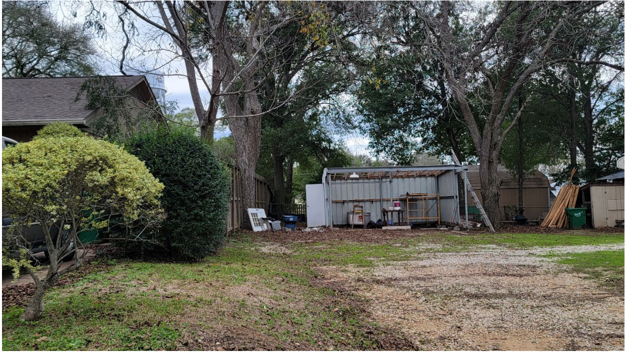
Existing metal storage shed to be removed.
