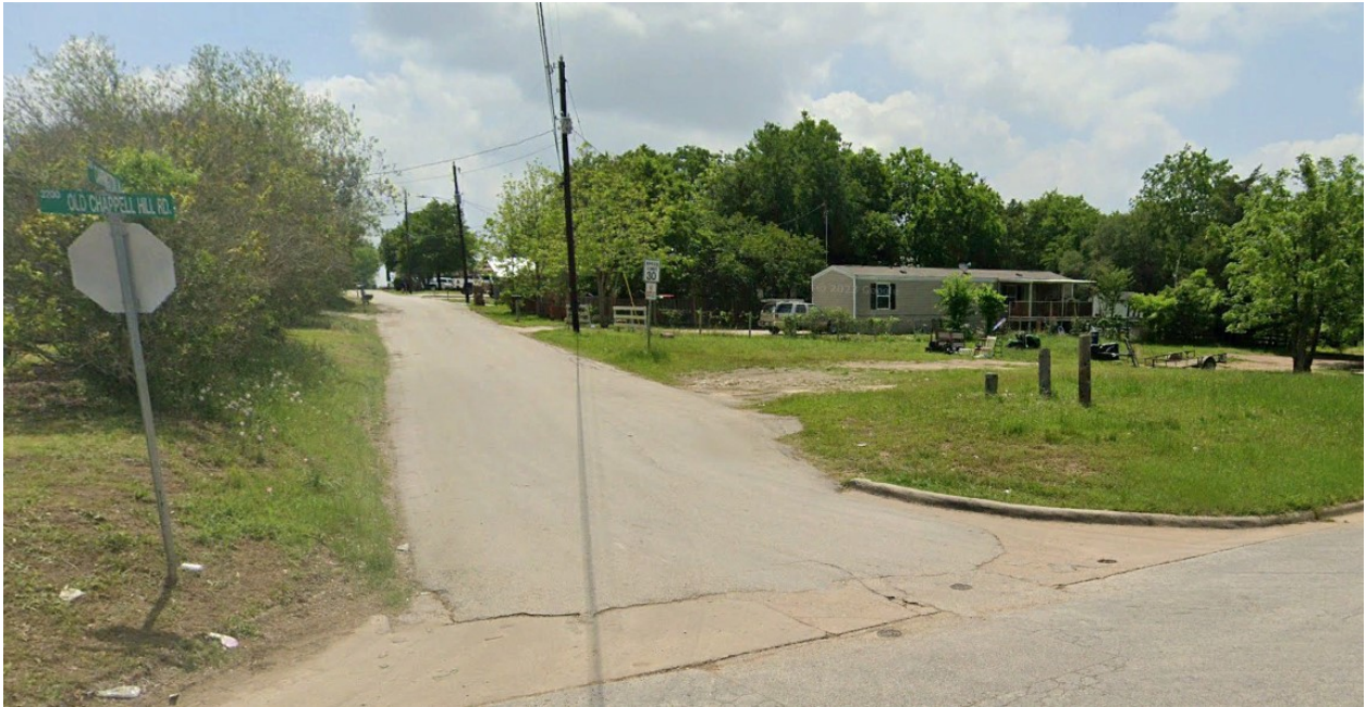
Carrington Lane (Before)
