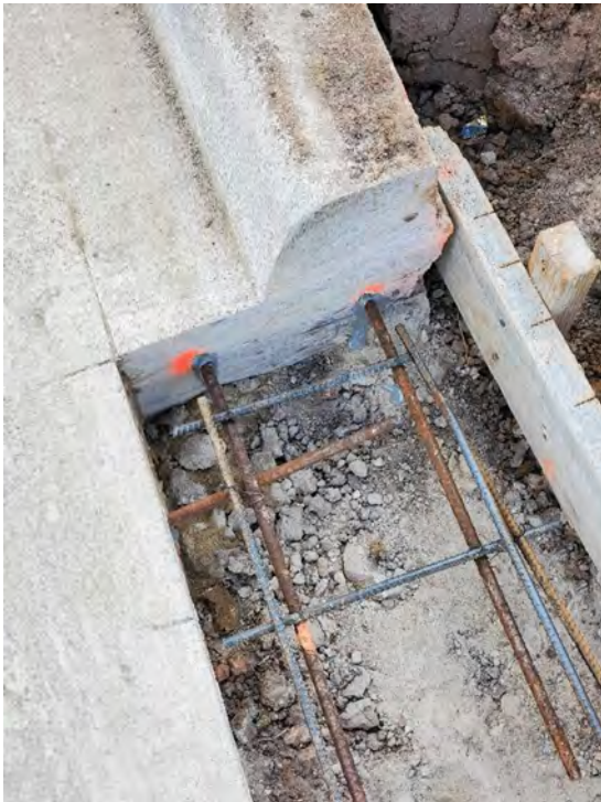
FIGURE 2 - REBAR DOWELED AND EPOXIED INTO EXISTING CURB
