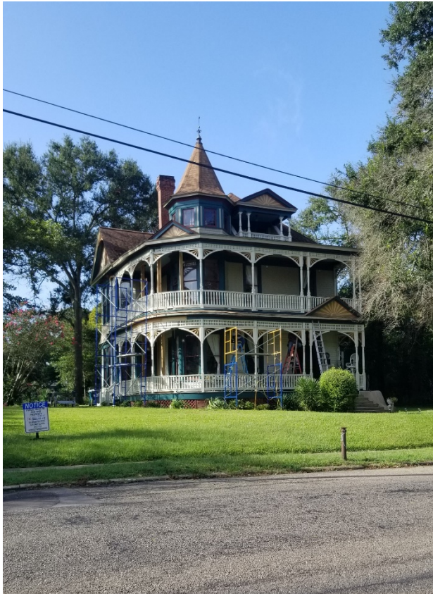
Principal Structure facing W. Alamo Street
