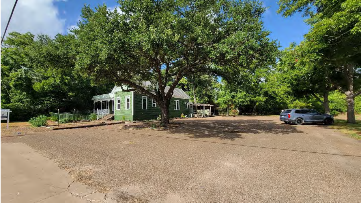
Subject Property Structure & Parking Area
