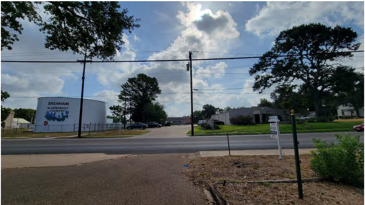
Water plant & Medical Offices to the East
