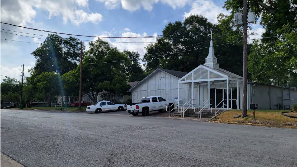
504 E 6 th Street and adjacent residential to the east
