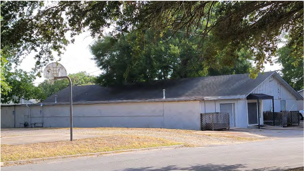
Rear of 504 E 6 th Street & parking area
