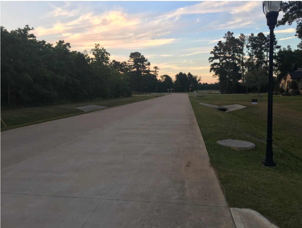
Concrete Pavement with Open Ditch Drainage
