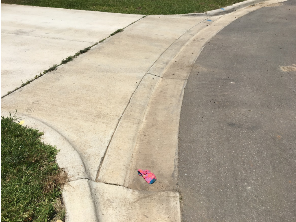
Concrete Curb and Gutter w/ Asphalt Pavement
