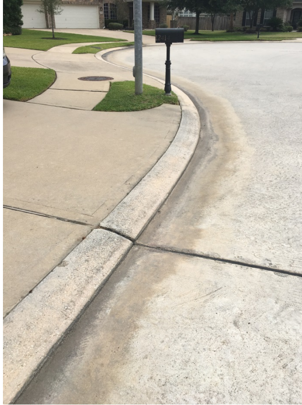
Concrete Laydown Curb and Gutter with Concrete Pavement
