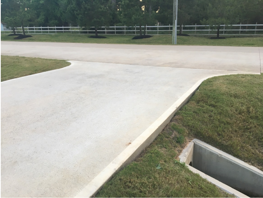
Concrete Pavement with Open Ditch Drainage
