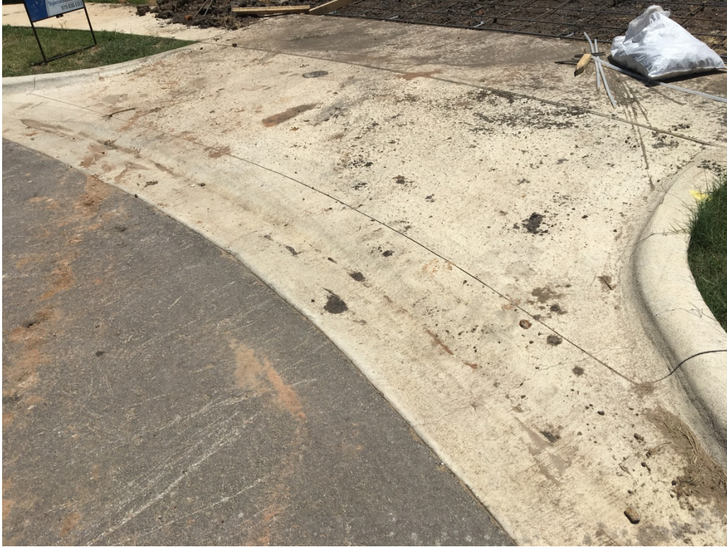
Concrete Curb and Gutter w/ Asphalt Pavement
