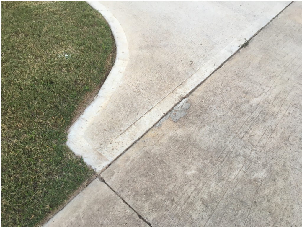
Concrete Pavement with Open Ditch Drainage
