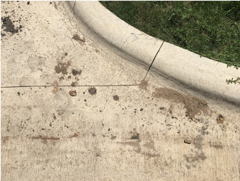
Concrete Curb and Gutter w/ Asphalt Pavement
