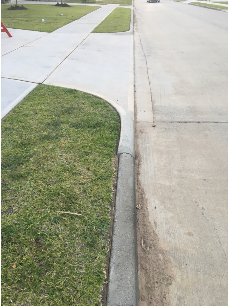
Concrete Curb and Gutter with Concrete Pavement and 6" Curb
