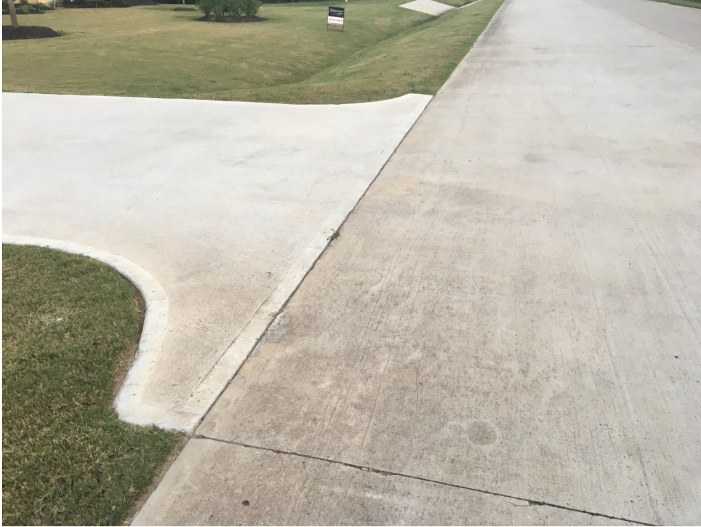
Concrete Pavement with Open Ditch Drainage
