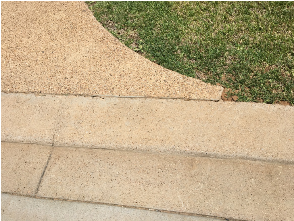
Concrete Laydown Curb and Gutter with Concrete Pavement
