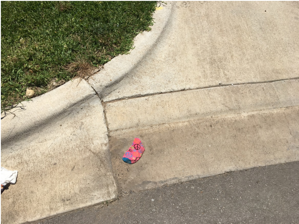
Concrete Curb and Gutter w/ Asphalt Pavement
