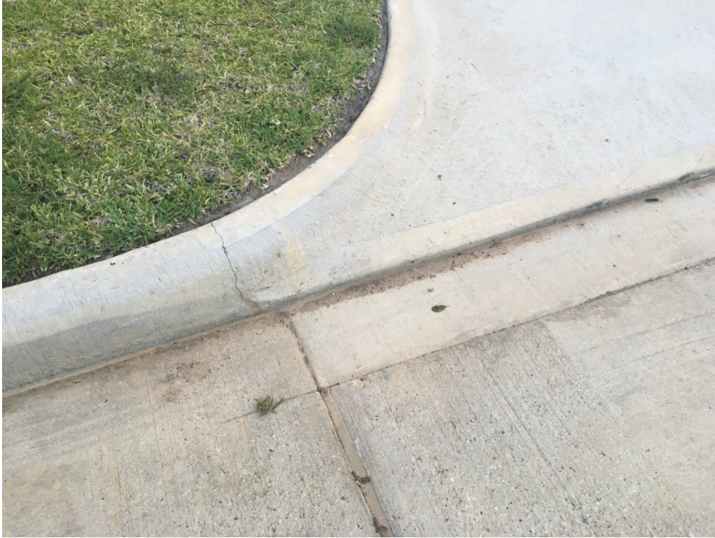
Concrete Curb and Gutter with Concrete Pavement and 6" Curb
