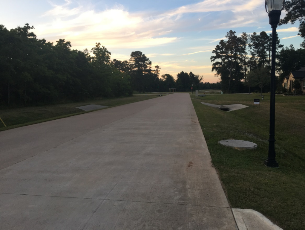
Concrete Pavement with Open Ditch Drainage
