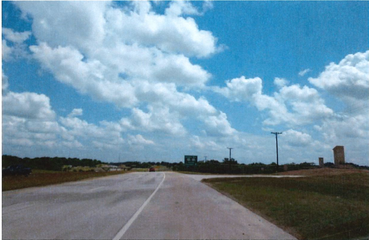
E1- SH 36 @ Vineyard Pass – southbound along SH-36
